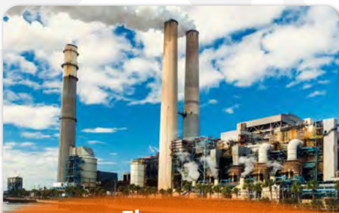
Flue gas desulphurisation systems
