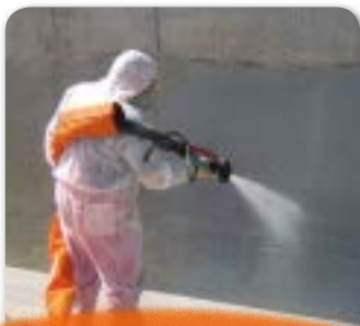
Mobile coating on-site
